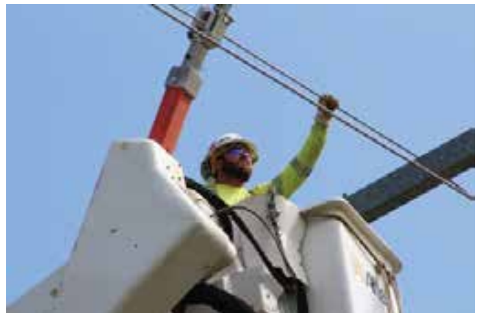
Job 1964-Ethan Nuttall transferring wire.
